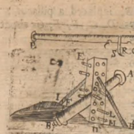
two supports, or props, *A B*, the Cannon; *O P*, the Lever, *S R* or *S*, the two notches in the Lever, and *Q*, *A* the hooke where the burthen or Cannon is tyed to. The rest of the operation is facill, that the youngest schollers or learners canhot fail to performe it: to teach *Minerva* were in vaine, and it were to Mathematicians injury in the succeeding Ages.
